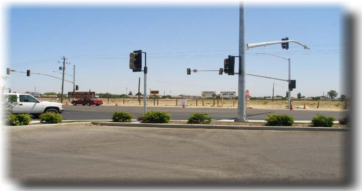
Traffic Signal Project at “B” Street and Winton Parkway
