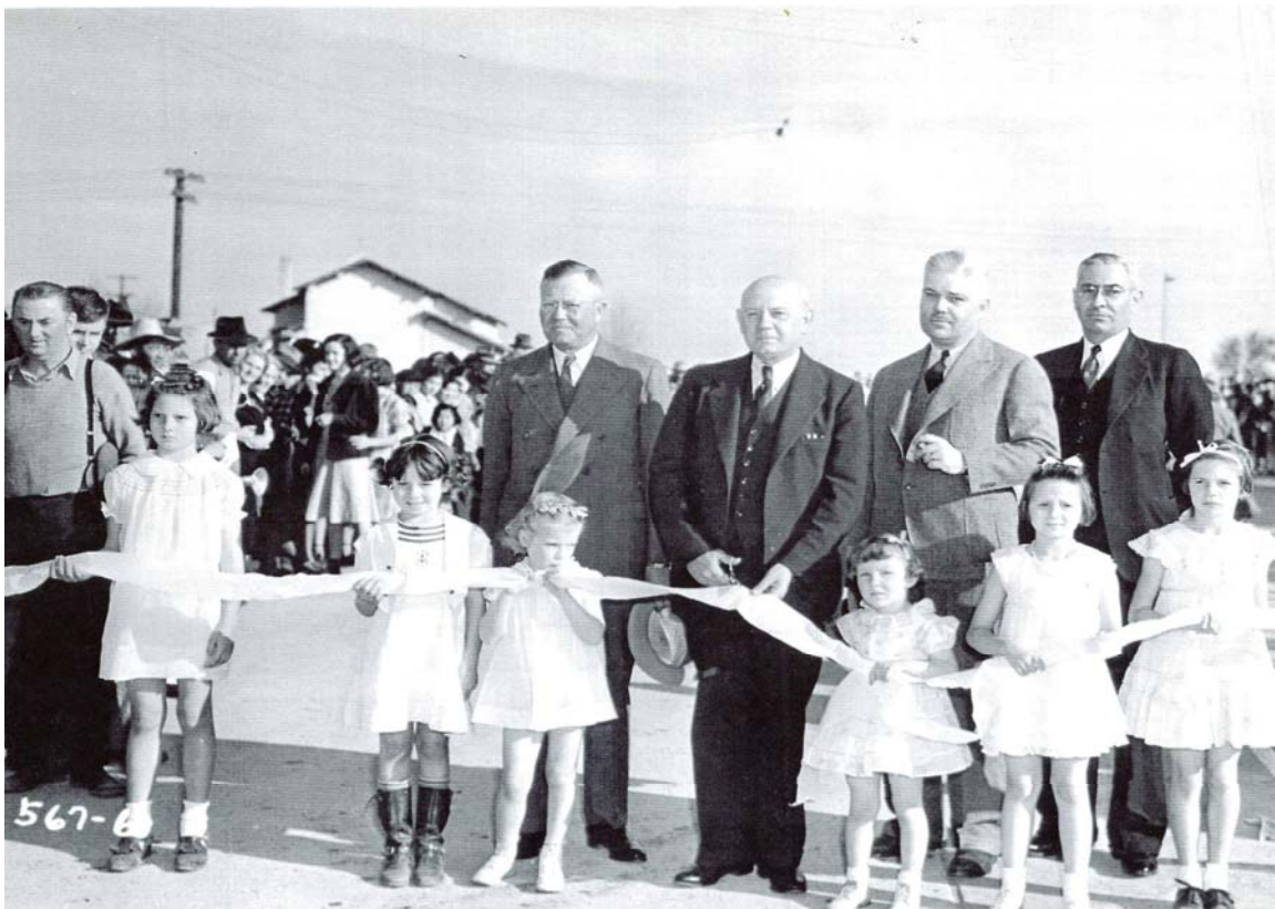
Opening of Underpass and Freeway Through Livingston--1939
